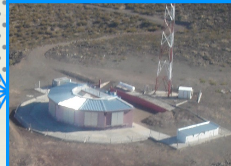
4 fluorescence detectors (24 telescopes up to 30°)
