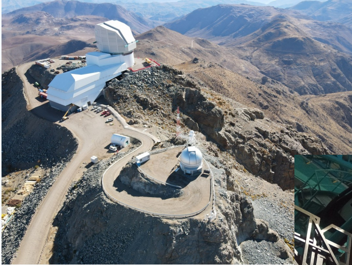
Dome almost 100% finished
