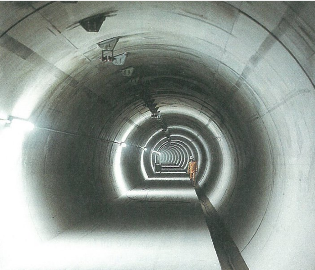
LEP tunnel before installation of bending magnets
