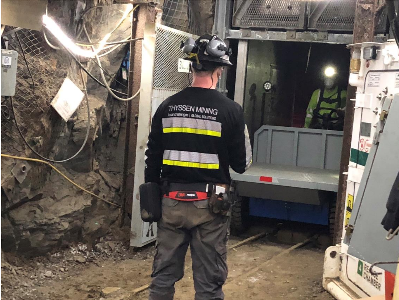
First underground equipment to arrive at 4850L: Shotcrete Transporter
