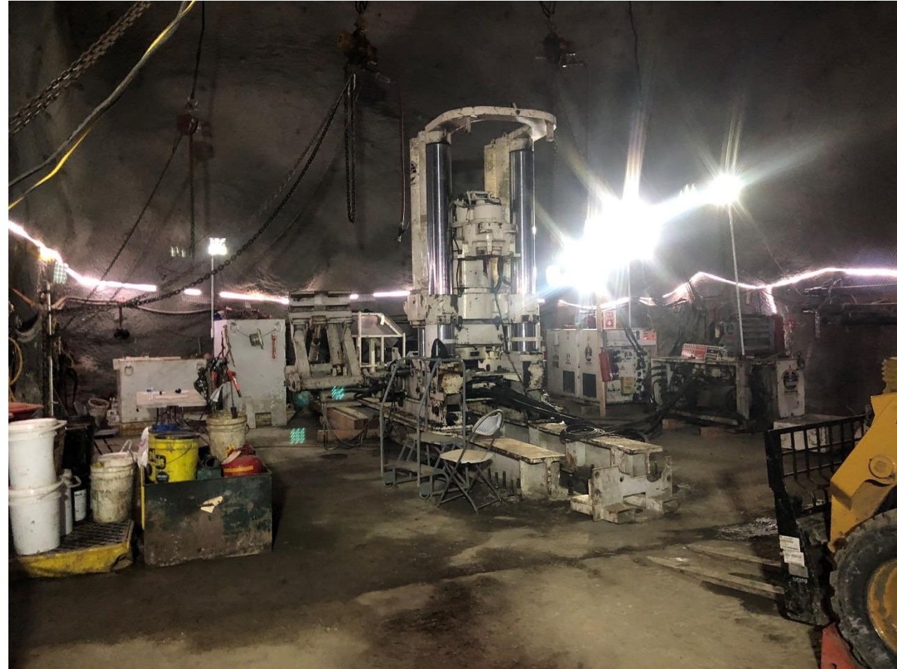
Raise Bore Machine being assembled in 3650L cavern
