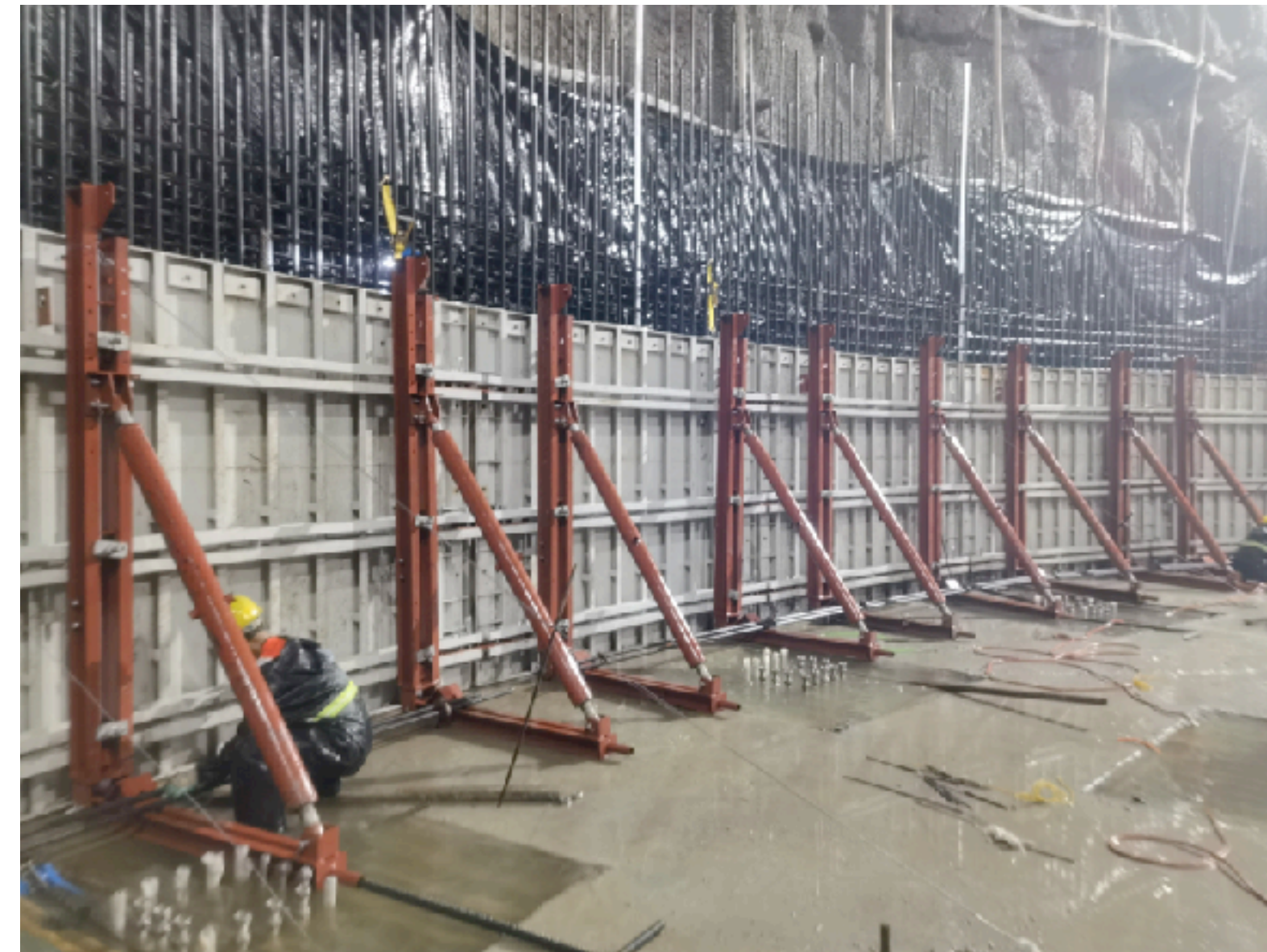
Preparation for side wall concrete, 15 April 2021
