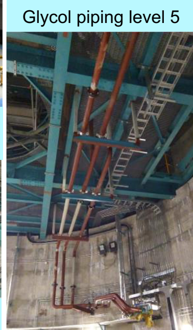
Cable trays & piping under TMA
