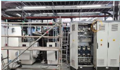
Oil supply pump level 1
