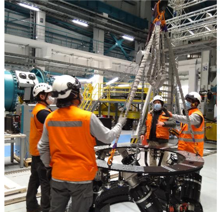
Team lifting Camera Hexapod/Rotator with bridge crane on 3 rd level
