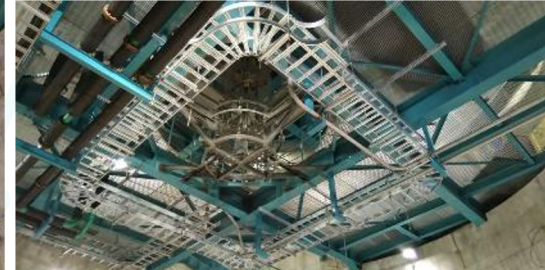
Cable trays & piping under TMA
