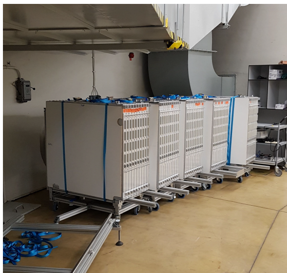
Detector dismantling started the 1st July
