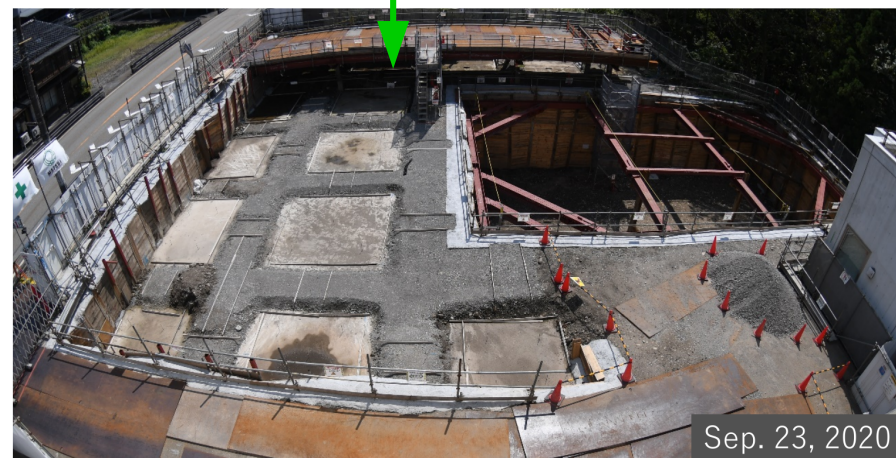
Construction of base structure is ongoing.
