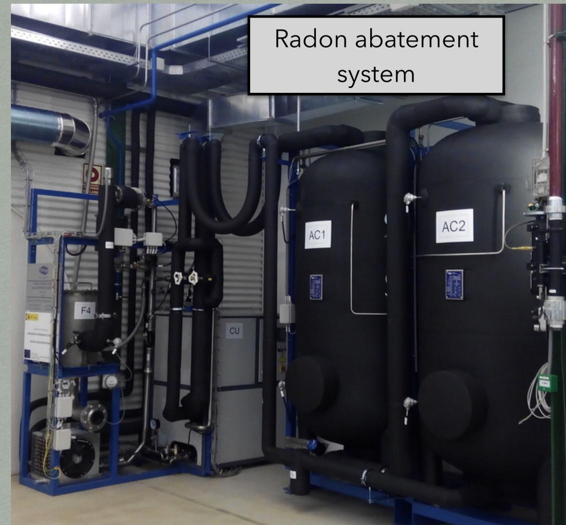
Backgrounds induced by airborne radon eliminated by providing Rn-free air to the NEXT shielding structure surrounding the vessel
