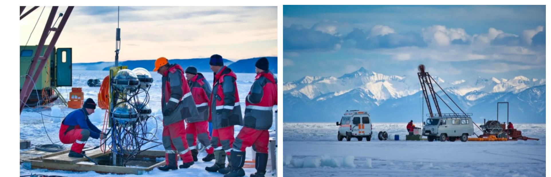
Fig. 2: Pictures of the installation of cluster 7 in lake Baikal
