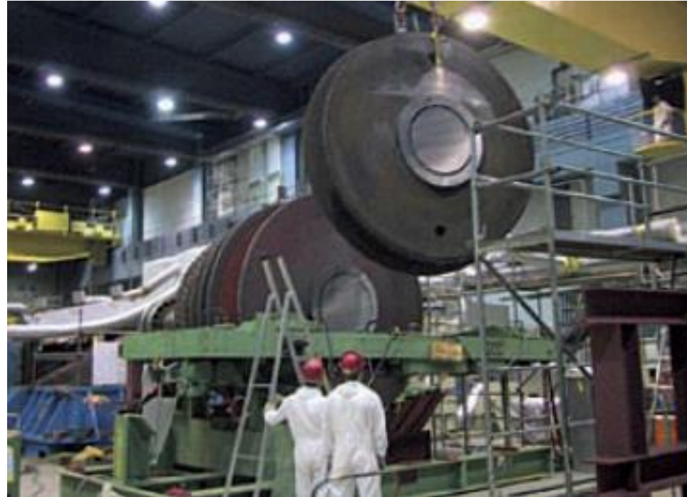
Dismantling the turbine
