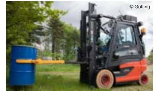
Removal of contaminated material
