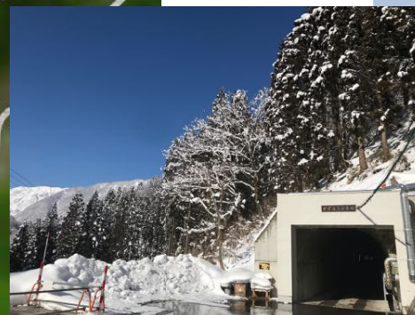
KAGRA Tunnel Entrance
