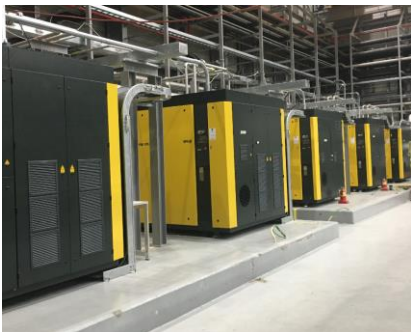
Compressors and Oil Removal System (WCS)
