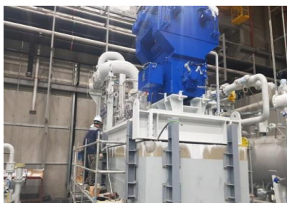
Compressors and Oil Removal System (WCS)
