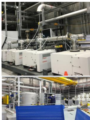
Compressors and Oil Removal System (WCS)
