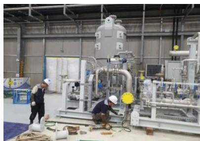
Compressors and Oil Removal System (WCS)
