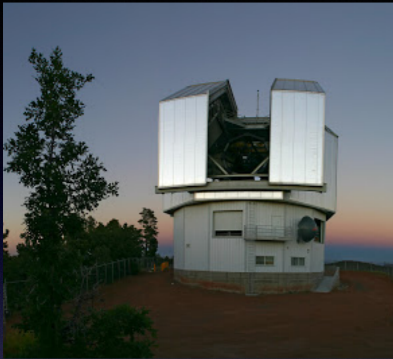
Discovery Channel Telescope (DCT) Arizona, USA
