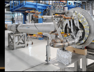
Cryo bypas line
