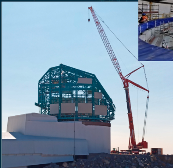
500 Ton crane reassembly this week for installation of trunnions in February.
