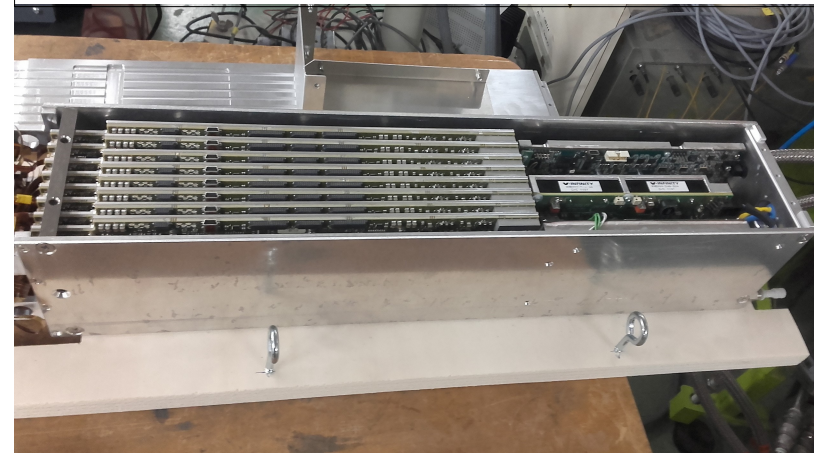
All mounted in the shelter
