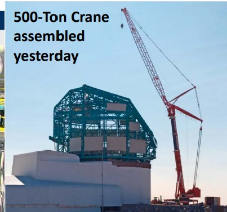
Telescope Mount in Assembly on Cerro Pachón
