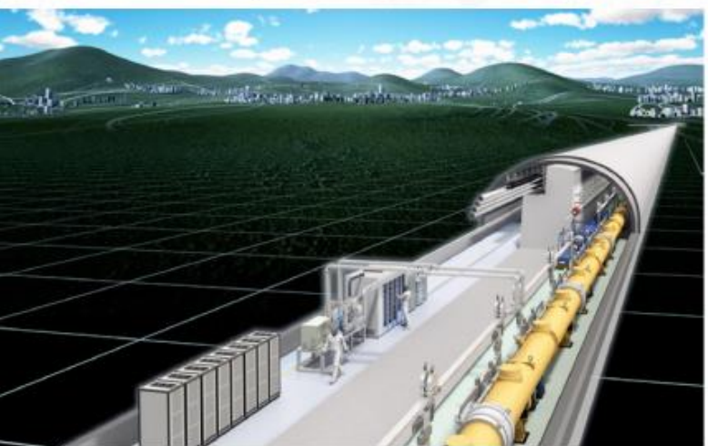
International Linear Collider (ILC): Japan \sqrt{s} : 250 - 1000 GeV, Now concentrating on \sqrt{s} = 250 GeV, Length: 21 km (250 GeV)
