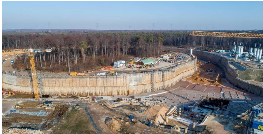
Excavation SIS100 tunnel
