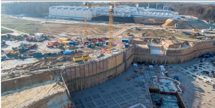
Excavation transfer building & CBM cave
