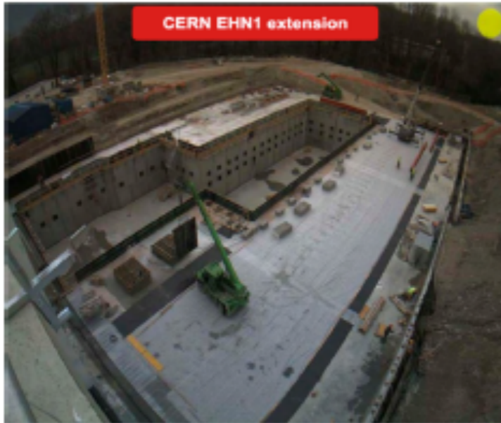
March 2016, construction of EHN1 extension
