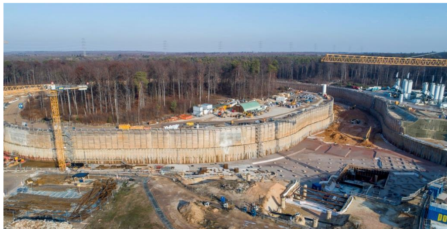
Excavation SIS100 tunnel
