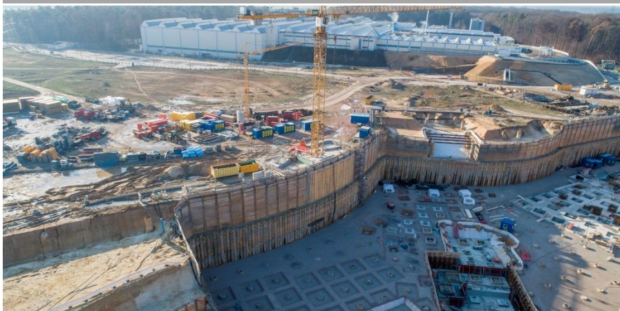
Excavation transfer building & CBM cave
