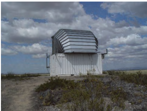
The LIDAR enclosure at Los Leones (Credit: Pierre Auger Observatory)
