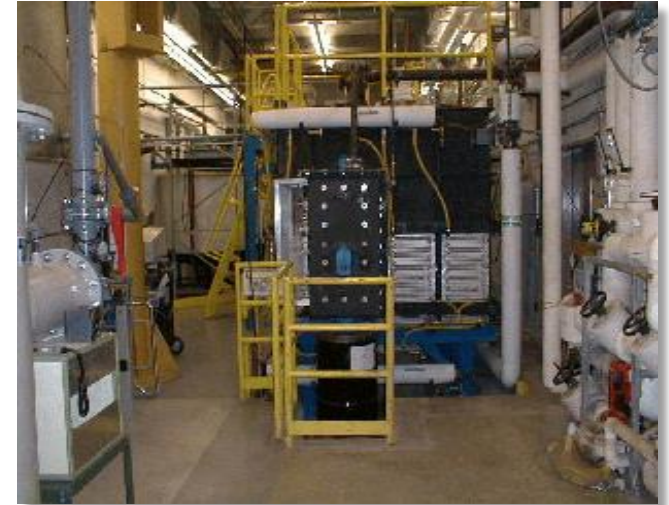
VSL DM1200 HLW Pilot Melter System
