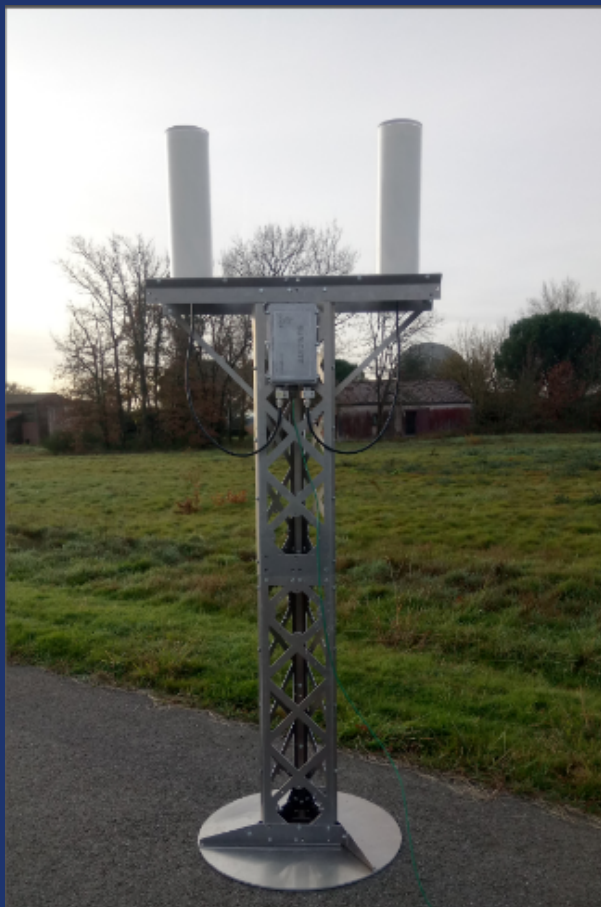
The VHF Ground Station
