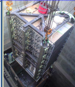
Beam dump completed
