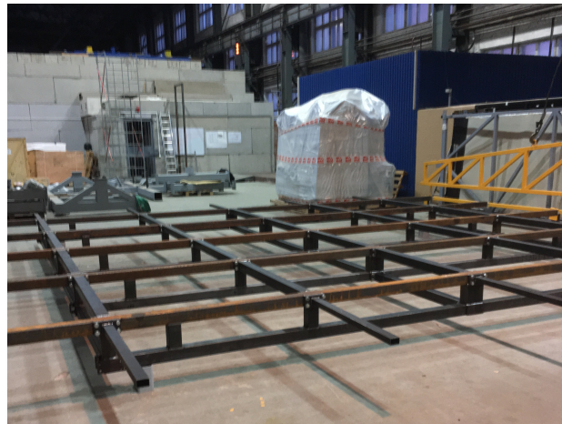
Wall Support structure
