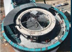
For Azimuth rails sectors installation
