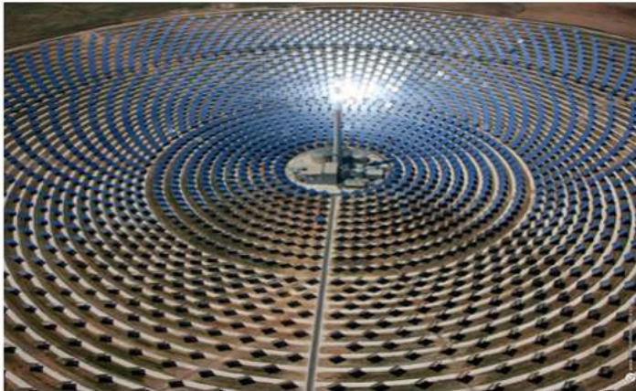
Tower power Plant (Gemasolar, Spain)
