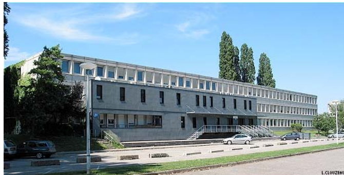
Figure 1: Nautibus building of the Université Claude Bernard Lyon1. 600 m 2 at the second floor will be dedicated to the EGI office.
