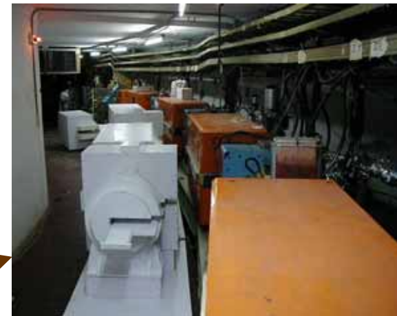
Two rings tunnel
