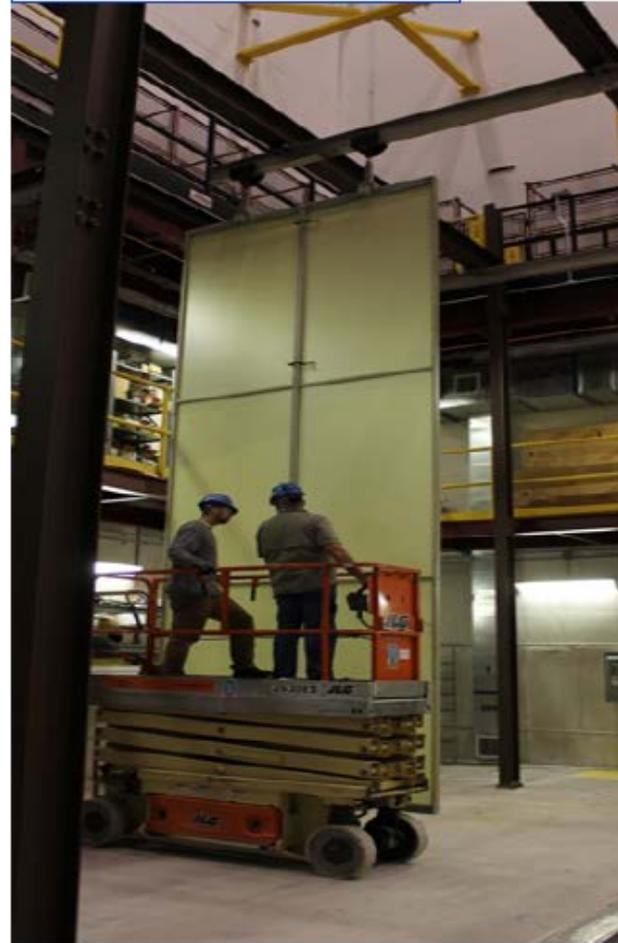
18 individual “panels” assembled into units of 3 and assemblies of 2 panels; 3 total panels needed
