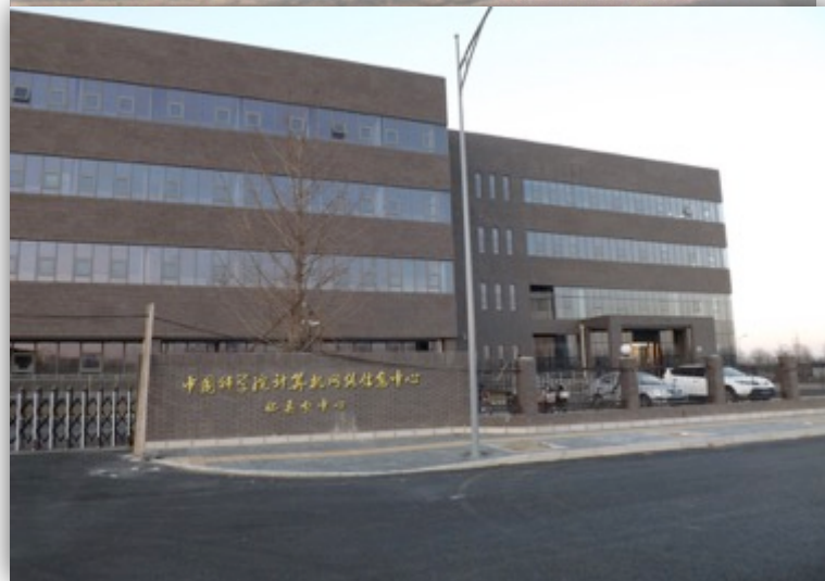
Data Center located in HuaiRou District, Beijing
