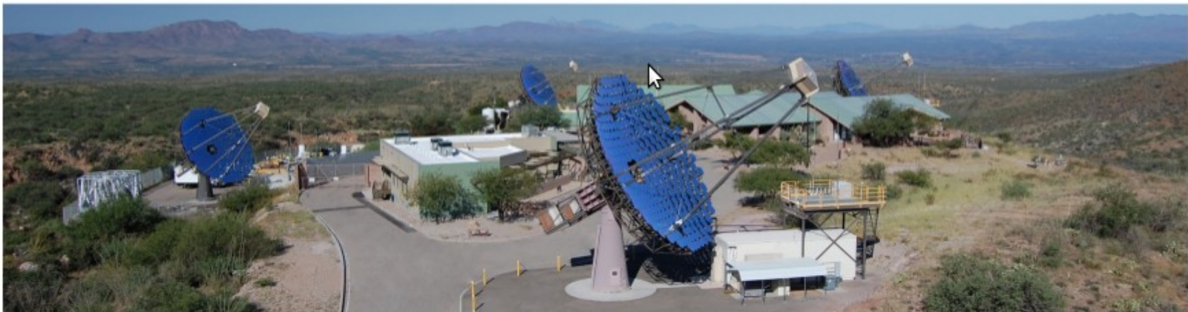
Figure 3.5.: Currently operating third generation IACT arrays: The MAGIC telescopes on La Palma, Canarian Islands ( upper left , mirror diameters 17 m), the four H.E.S.S. telescopes (mirror diameters 12 m) and the large H.E.S.S. II telescope (average mirror diameter 28 m) on the Khomas Highland in Namibia ( upper right ), and the VERITAS array near Tucson, Arizona, USA ( bottom , mirror diameters 12 m). Image credits by the MAGIC/H.E.S.S. & VERITAS collaborations.
