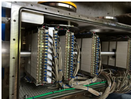
Five first Guard Ring stations during installation
