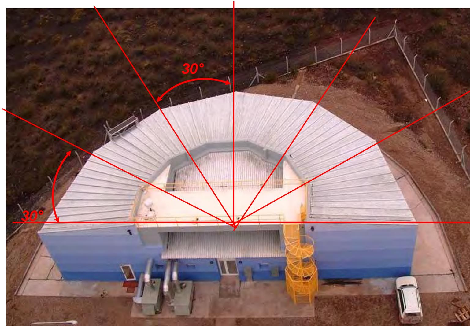
*6 telescopes, each with  $30^\circ \times 30^\circ$  FOV*
