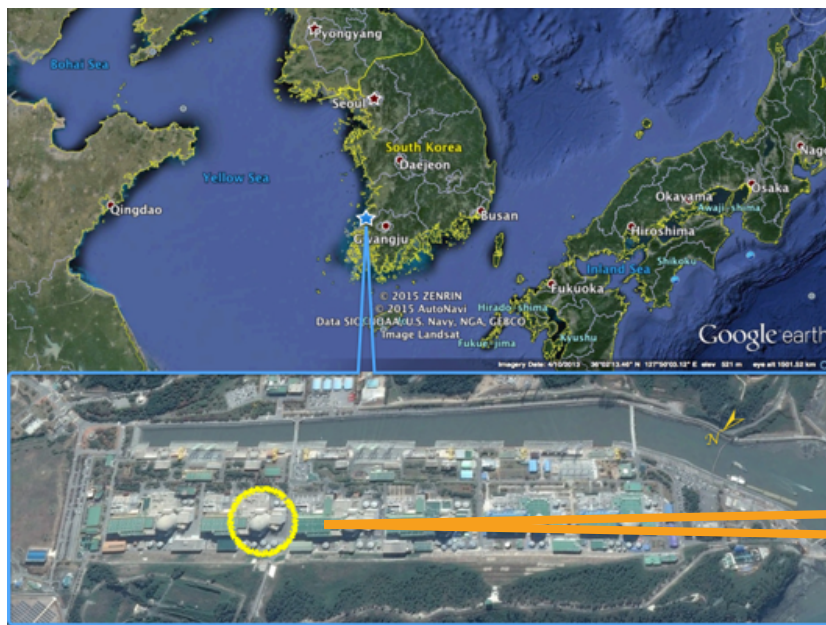
Reactor Unit 5, Hanbit NPP in Younggwang, Korea (Reno Site)
