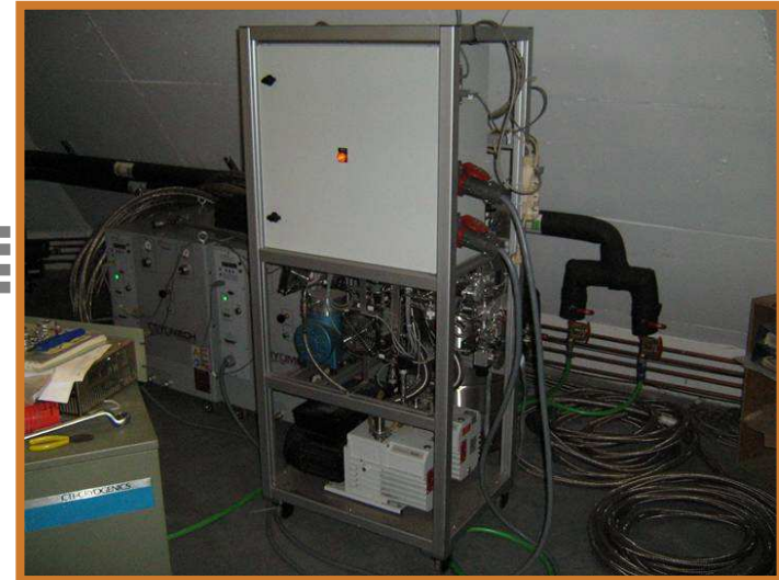
The dilution gas handling in the basement
