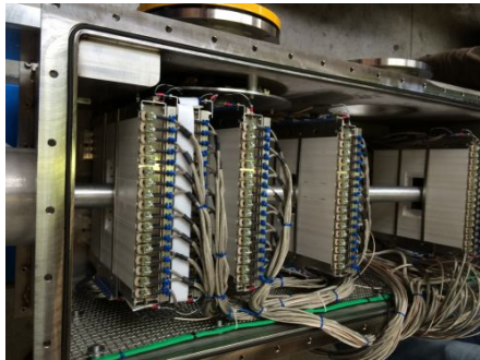
Five first Guard Ring stations during installation
