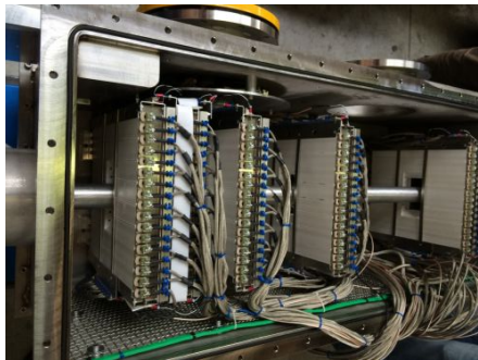
Five first Guard Ring stations during installation
