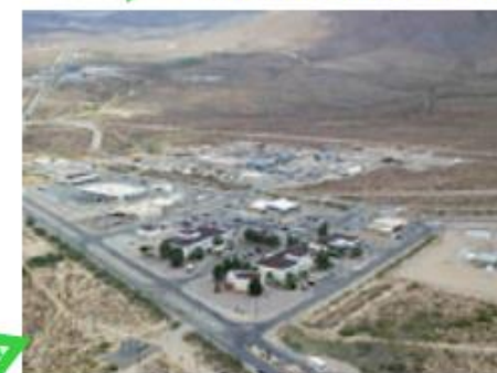
White Sands Ground Terminal, NM
