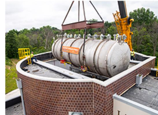
The 30-ton MicroBooNE neutrino detector is gently lowered into the Liquid-Argon Test Facility at Fermilab on Monday, June 23. The detector will become the centerpiece of the MicroBooNE experiment, which will study ghostly particles called neutrinos. *Photo: Fermilab*
