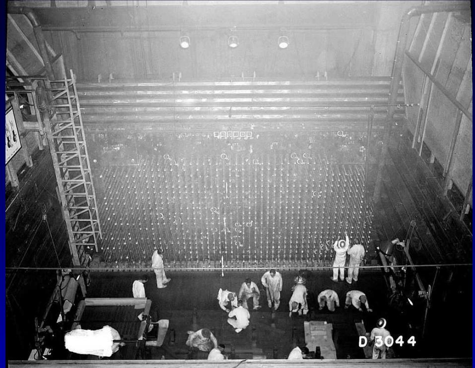
Hanford, B reactor, making plutonium for the Trinity device and Little Boy
